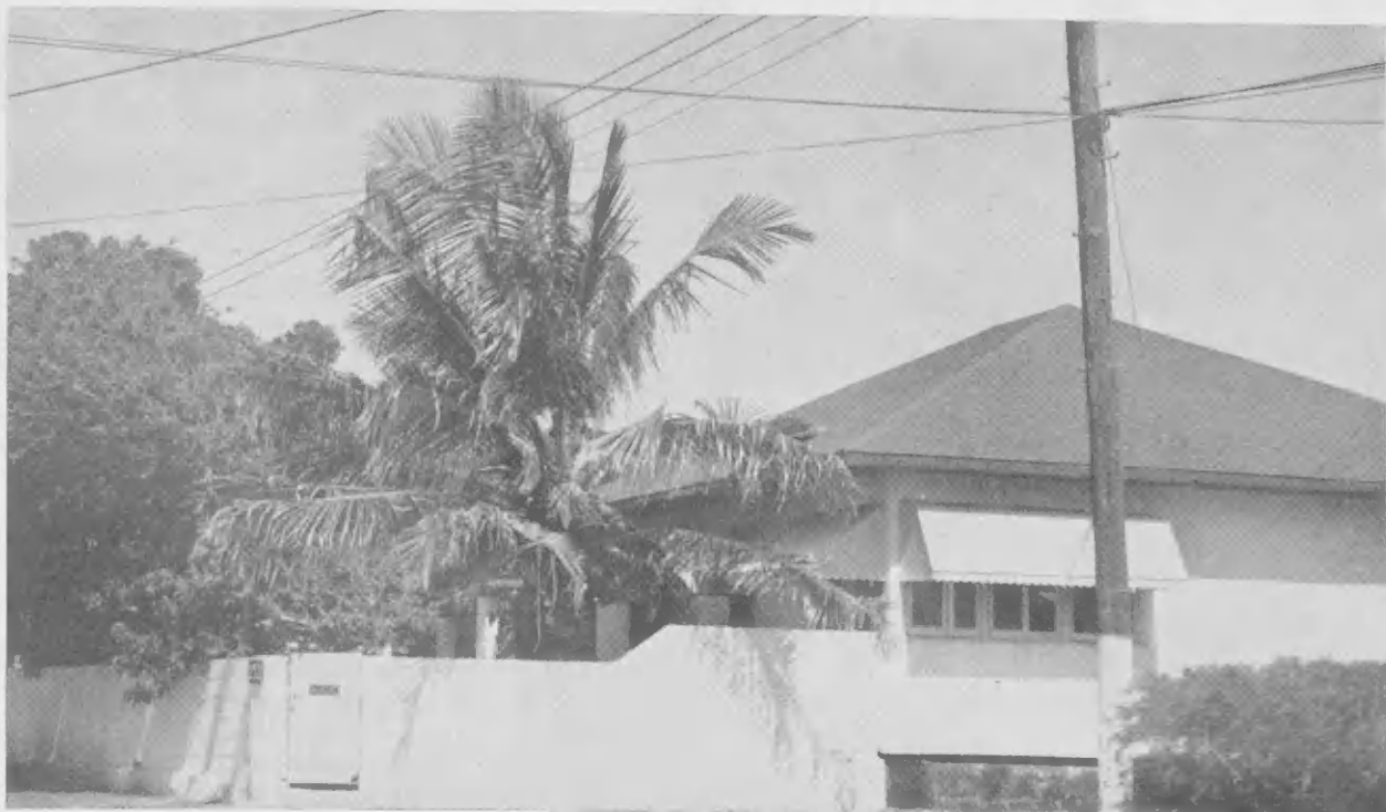
ELECTRIC WIRES entangled in trees are like WAYA ELECTRICO cu ta pasa den palu ta mescos cu enemigo scondi.
